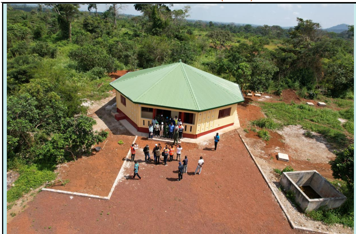
Figure 48: Rehabilitation/completion of the Mount Nimba Nature Conservancy Base (©UNOPS).
